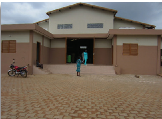
Ikpilè boasts a 1,000-ton Gari Warehouse
