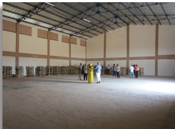
A committee tours the inside of the Ifangni 1,000-ton Maize Warehouse
