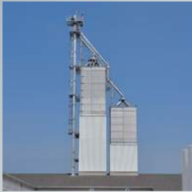
| Tower Blend Systems
